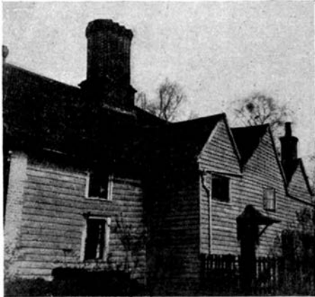
NEW HOUSE FARM, GREENSTED, ESSEX
